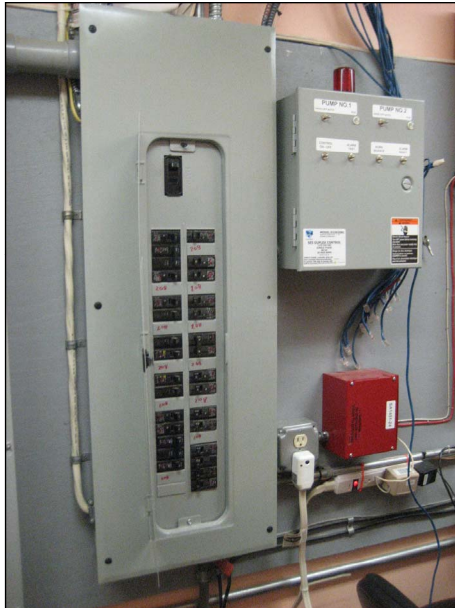
Photograph 6: Air handling breaker switches and control circuitry.
